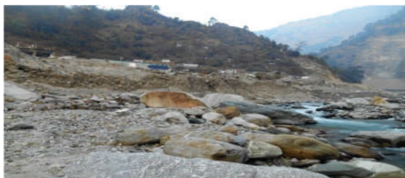
Eroded bank of Mandakini Valley after Kedarnath flood
