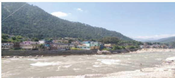
Flood protection work carried out in Mandakin valley
